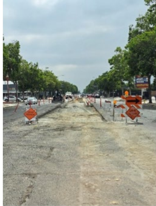
Holt Avenue Median Construction
