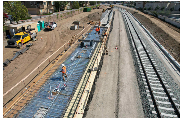
Crews constructing the platform for the future Glendora station
